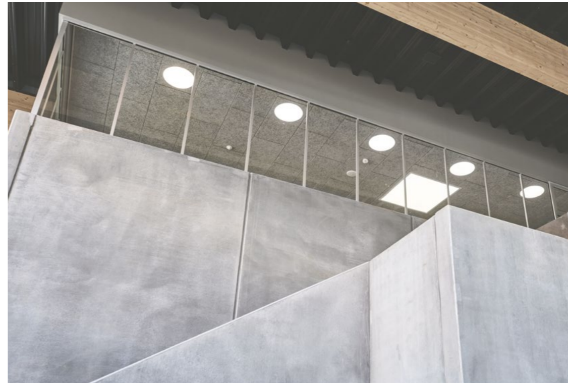
TRIPLAN LITE® | EI 60. Junction with transoms
