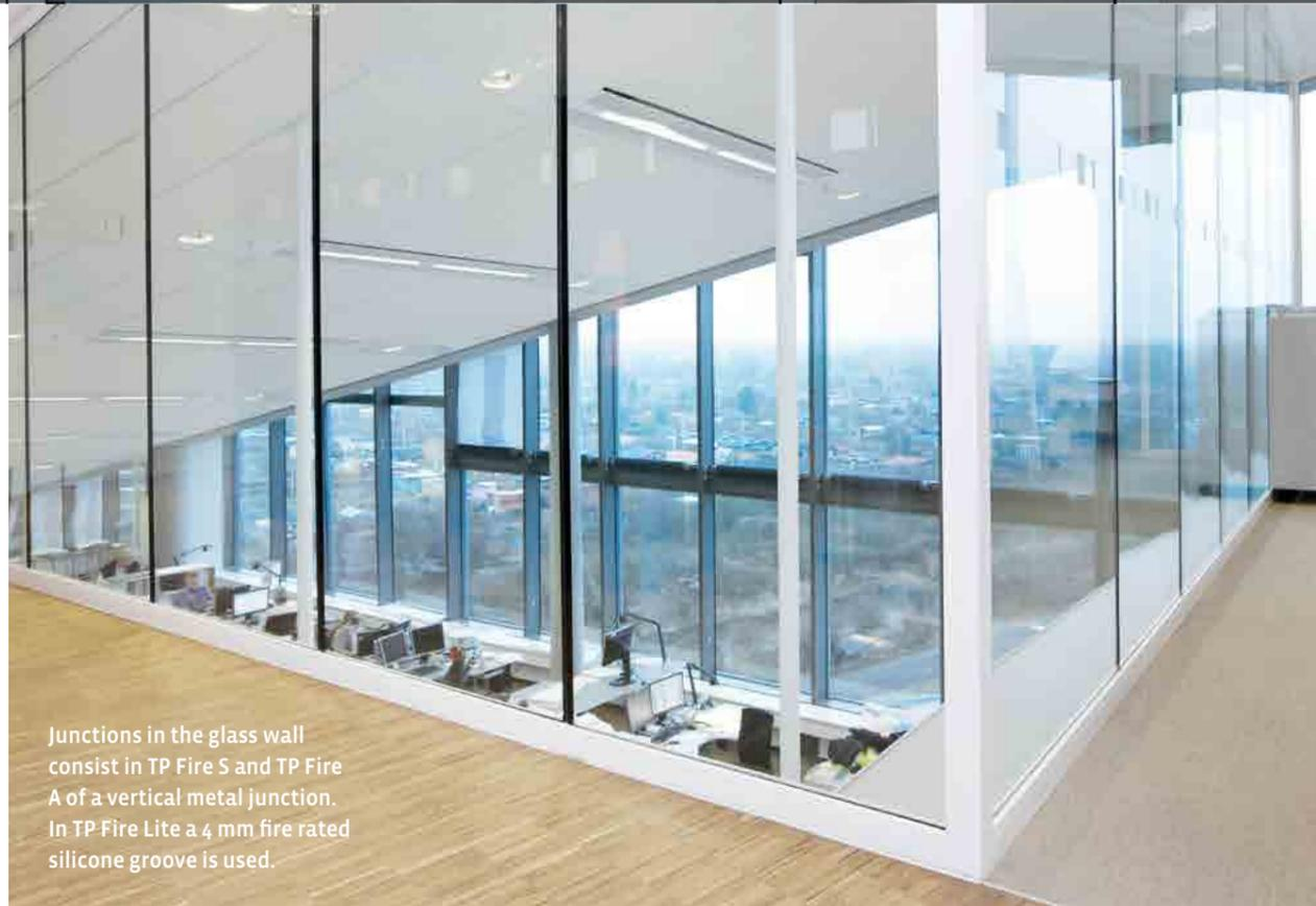
Junctions in the glass wall consist in TP Fire S and TP Fire A of a vertical metal junction. In TP Fire Lite a 4 mm fire rated silicone groove is used.
