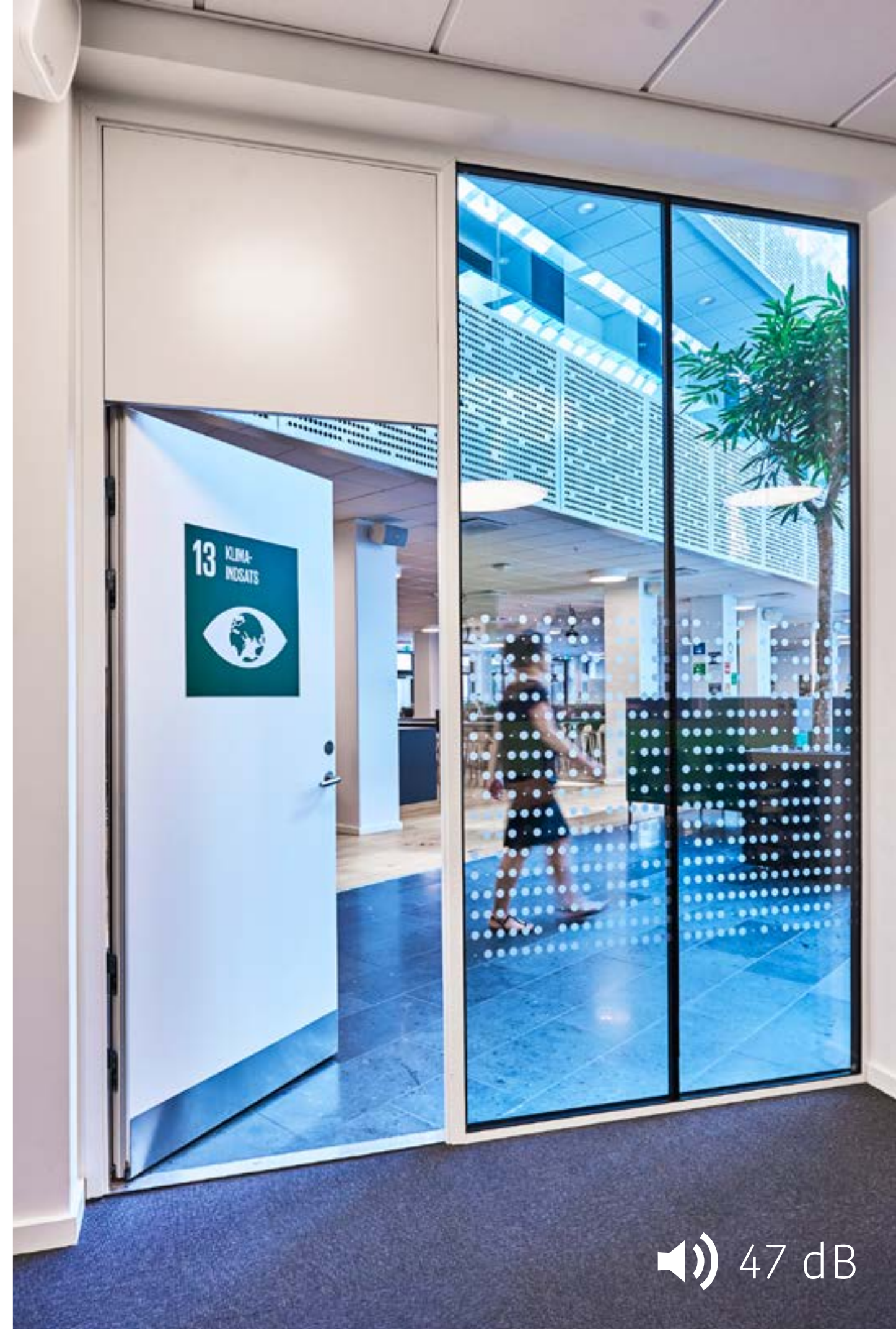
SOUND RATED GLASS | TAPED JOINT | 40 DB SOLID DOOR WITH OVERPANEL | WHITE FRAMING
